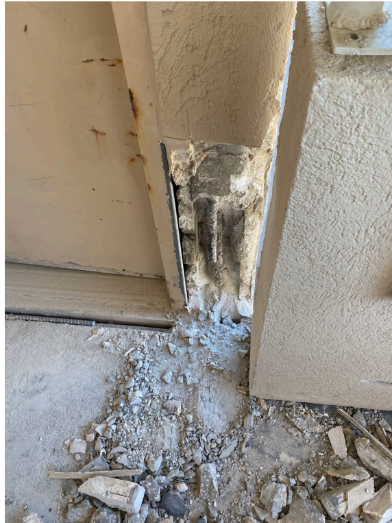
Picture 1: In-progress wall repair by North stairwell 7 th floor
