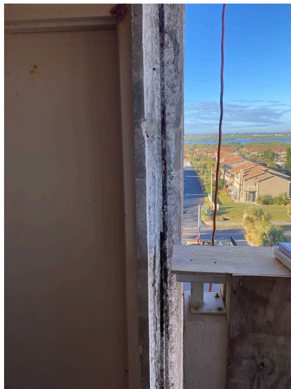
Picture 2: In-progress wall repair by North stairwell 6 th floor
